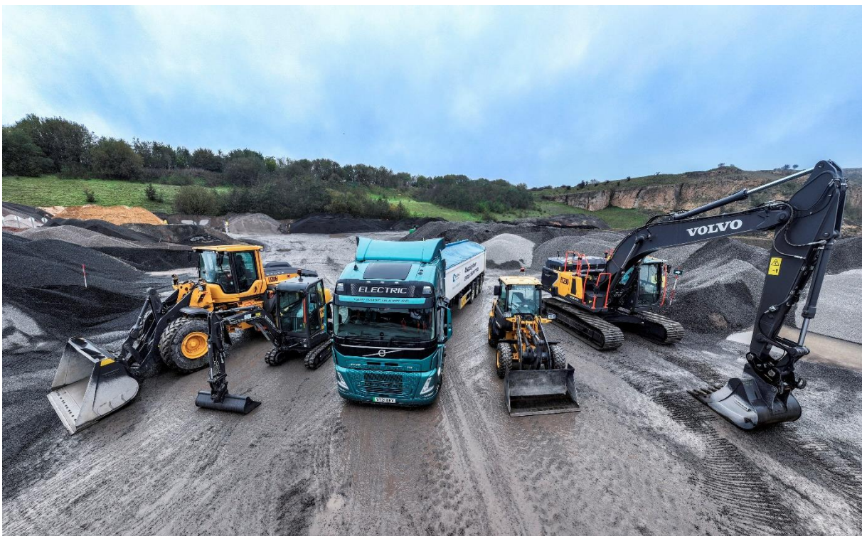
Zero-emission solutions by Volvo CE and Volvo Trucks on site in Durham, UK, with CRH company Tarmac
